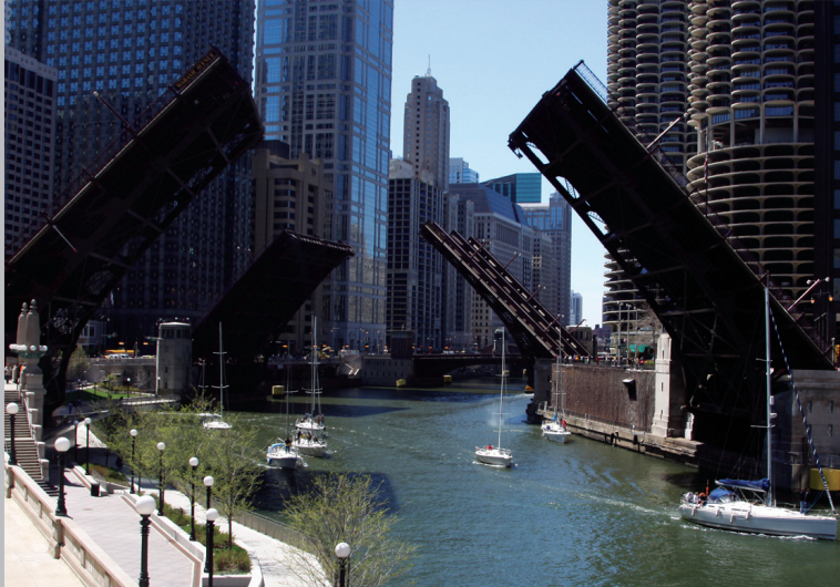
Bascule Bridges at Chicago River
